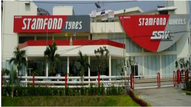
SSW wheels manufacturing factory, Nonthaburi
